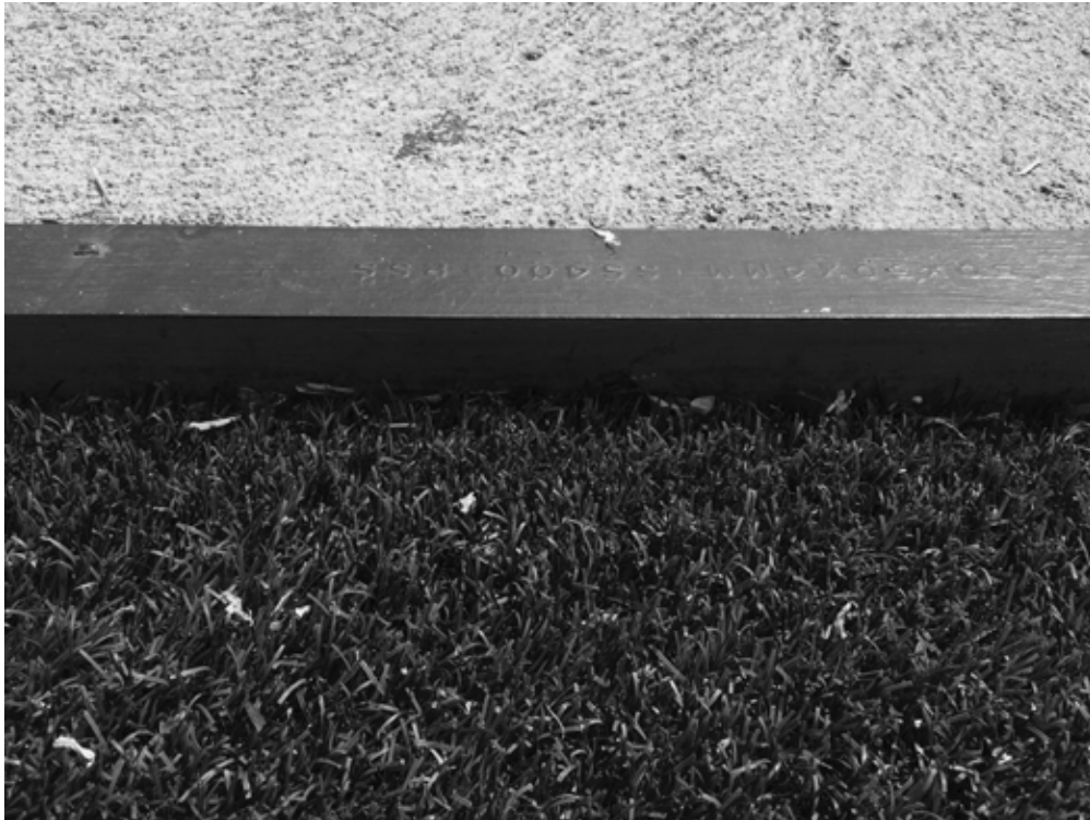
Figure 3 Concrete covered with metal sheet steel along the positions where hit by the wheelchair.
